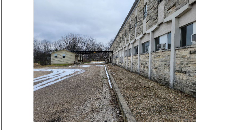
North wall of hospital and residential structure. Facing east.
