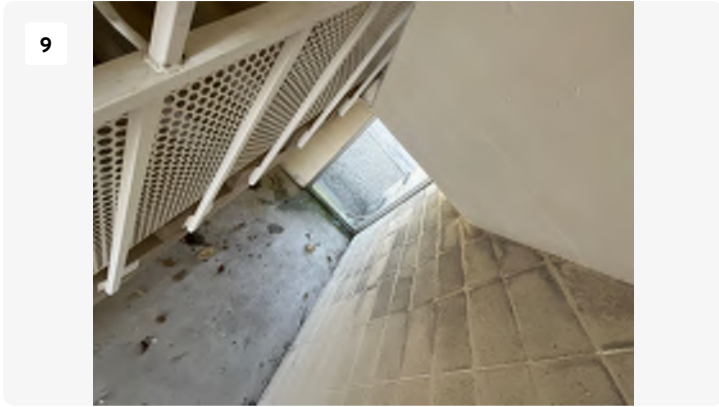
Project: Blackstone-hospital Date: 3/11/2024, 10:01am Creator: Logan Drake Tags: west stairwell to 2nd
