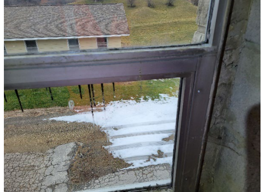
North half of second floor of the Subject Property facing west. Modern aluminum window with dripping window glazing on the north wall of the second floor northern room.
