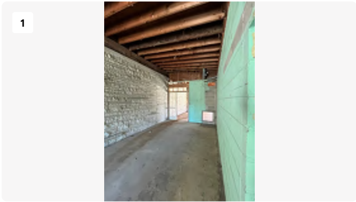
Project: Blackstone-hospital Date: 3/11/2024, 10:24am Creator: Logan Drake Tags: Garage Entry
