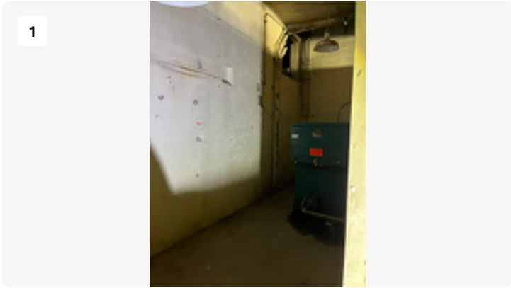
Project: Blackstone-hospital Date: 3/11/2024, 11:03am Creator: Logan Drake Tags: 1st floor Mechanical
