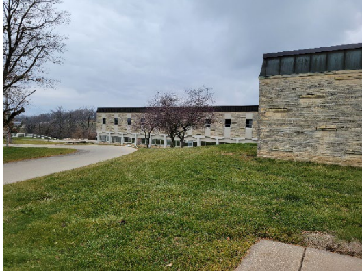
South side of the Subject Property, facing northwest.
