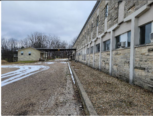
Southeast corner of the Subject Property, facing east. Building on the left was indicated as the nun's house.
