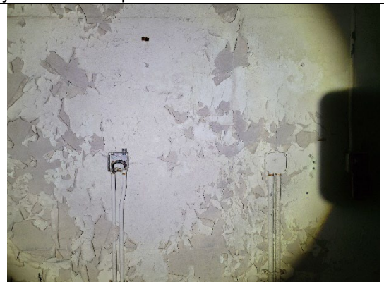
Power to the elevator mechanism. Out of picture is a Sump directly beneath the power switch.
