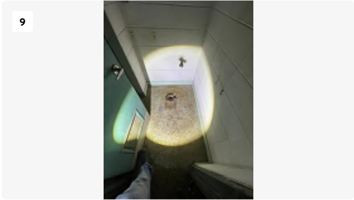
Project: Blackstone-hospital Date: 3/11/2024, 11:45am Creator: Logan Drake Tags: Rm 128 Mens Restroom 1st floor
