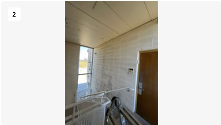
Project: Blackstone-hospital Date: 3/11/2024, 10:01am Creator: Logan Drake Tags: west stairwell to 2nd
