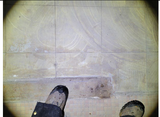
Vinyl floor tile on the second floor in the main room with mastic on top of the tile.
