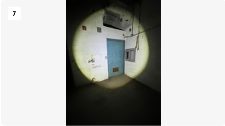
Project: Blackstone-hospital Date: 3/11/2024, 11:18am Creator: Logan Drake Tags: Rm 125 E Laundry
