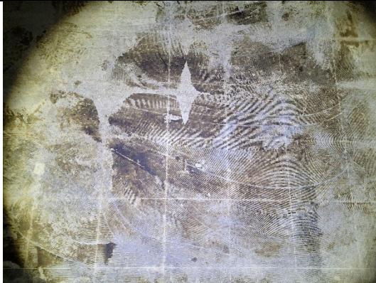
Vinyl floor tile on second floor within the main entrance.
