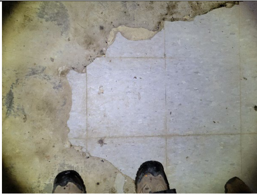
Multiple tiles on top of one another on the second floor in the main room.
