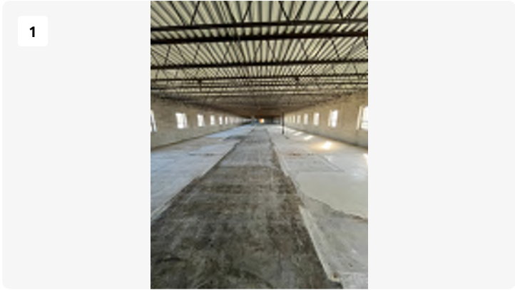
Project: Blackstone-hospital Date: 3/11/2024, 10:04am Creator: Logan Drake Tags: 2nd floor North open
