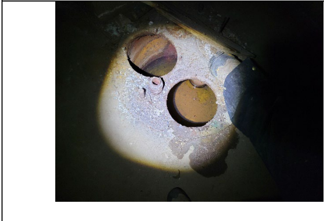
Sump in the diesel generator room.
