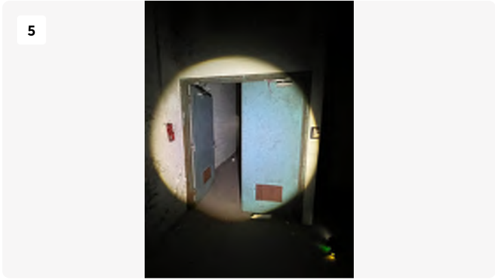
Project: Blackstone-hospital Date: 3/11/2024, 11:18am Creator: Logan Drake Tags: Rm 125 E Laundry
