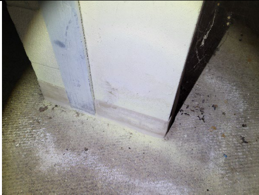
Corner outside of stairwell from second floor to first floor. Showing cove base, carpet, and sheetrock walls.
